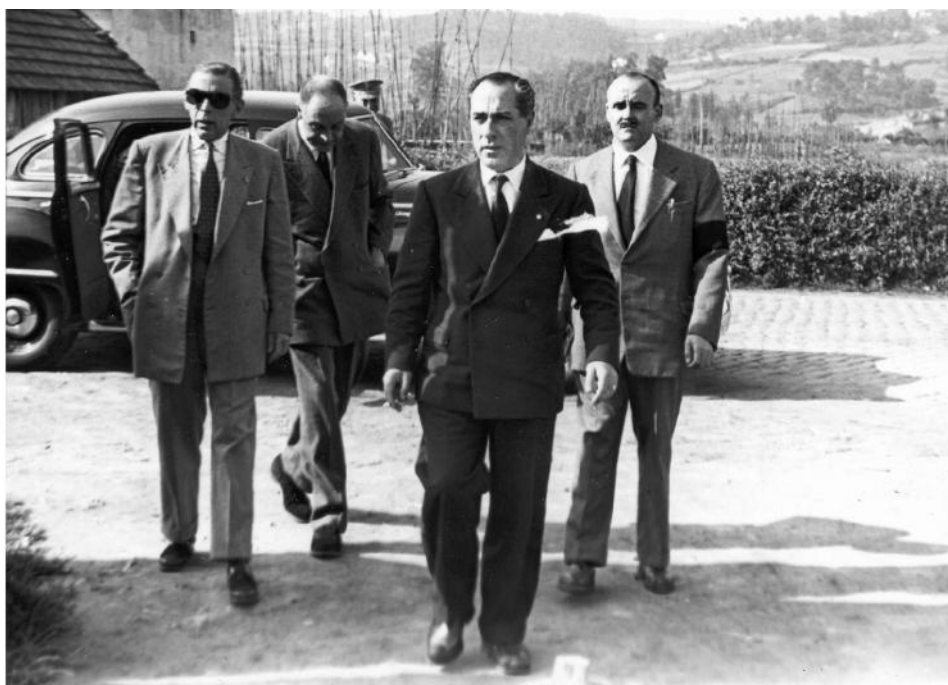
O Director Xeral, Rodríguez de Valcarcel, visitando as obras do antigo Instituto.
